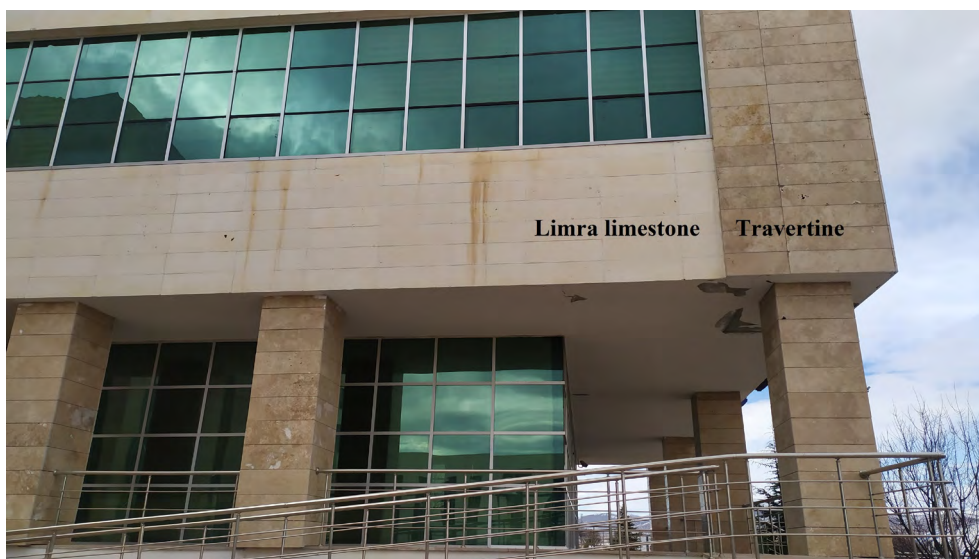
Fig. 1. View of a building where limra limestone and travertine are used as exterior cladding (Kırşehir Ahi Evran University)
